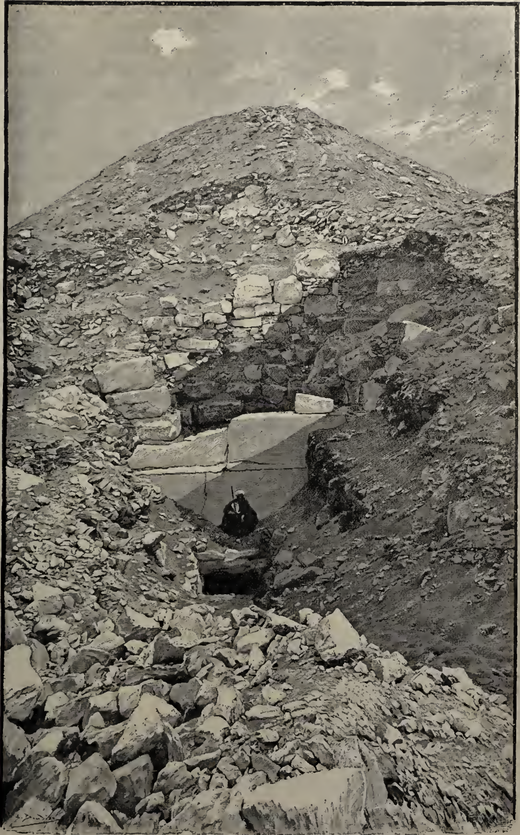
THE ENTRANCE TO THE PYRAMID OF UNAS AT SAQQARA. Drawn by Boudier, from a photograph by Emil Brugsch Bey.
